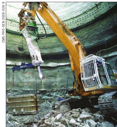
Fig. 1. A number of events occurred during construction that necessitated amendments to the LHC contracts. During construction of the ATLAS caverns and access shafts (left), the design of a vault using reinforced concrete beams was found to be technically unacceptable and had to be replaced. During excavation at the CMS site (right), meanwhile, the discovery of unforeseeable ground conditions required significant changes to the approach and led to the submission of disputes to an adjudication panel. In all cases, they were successfully resolved.
