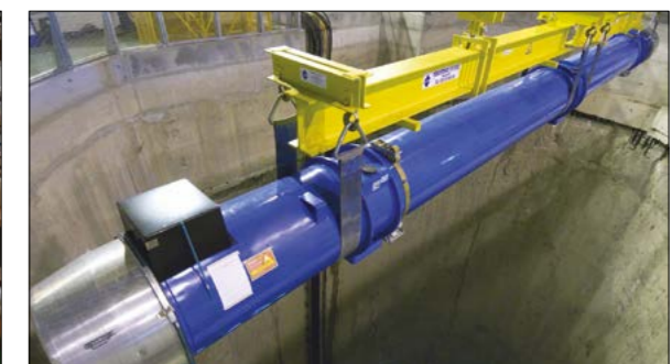
Fig. 2. The main components and tooling required to assemble the LHC dipole cold-masses were purchased by CERN and delivered to contractors (left, showing cold masses at German company Noell in 2003), who would then return the assembled cold masses to CERN for final insertion into the vacuum vessels (right, showing the final dipole being lowered into the LHC tunnel in April 2007). This approach was also applied to the superconducting strands and cables, the quantities of which were so huge that all major European manufacturers, as well as one US and one Japanese firm, were involved.
